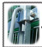
ALWAYS MAKE SURE THAT YOUR CAGE HOOKS ARE CORRECTLY POSITIONED
